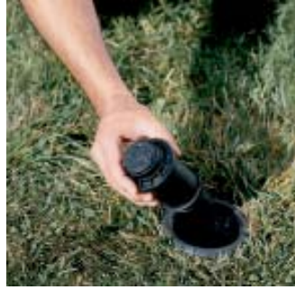
2. Thread entire ATR body/riser into canister.
