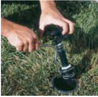
1. Remove internal assembly of existing sprinkler.
